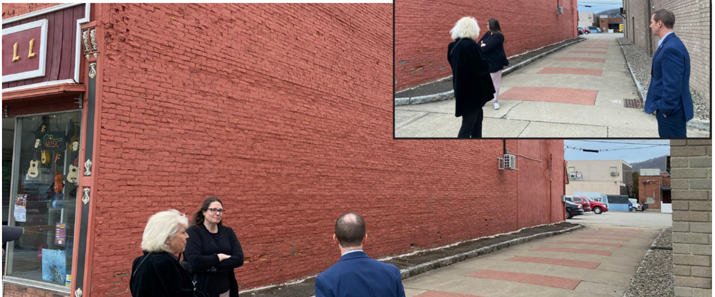
Existing conditions (before proposed alley improvements)
